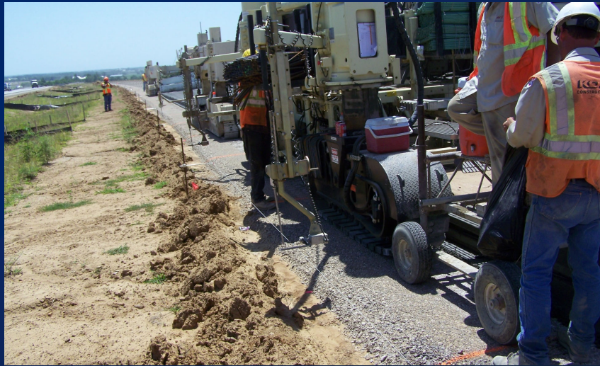
Inspectors checking different parts of the paving train
