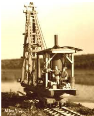
Railroad Steam Pile Driver 1912
