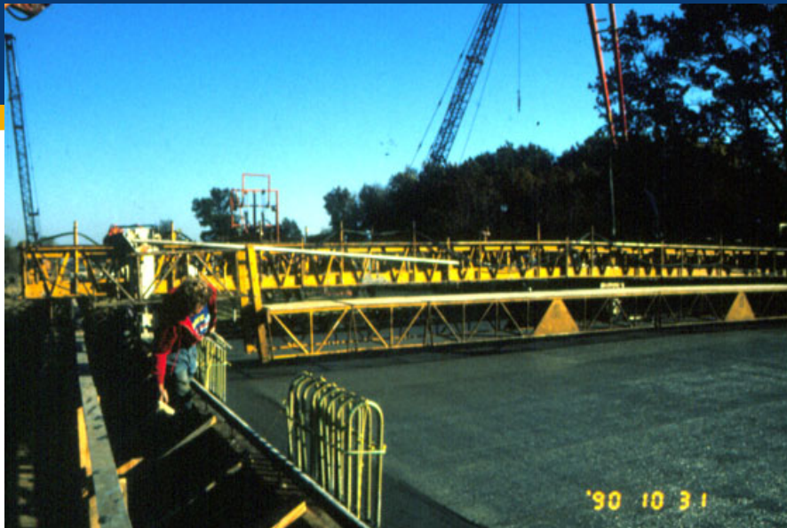
Float Train c. '90 (Transverse Grooving now done by multi-blade diamond abor, see Sub-Sec. f., p. 700-46)
